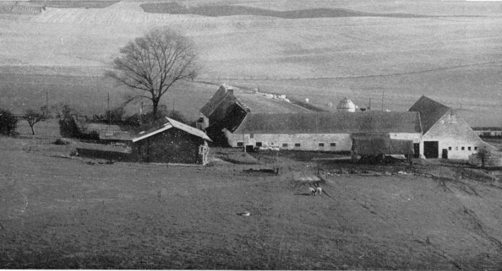
28. La Haye Sainte from the west. This photograph and numbers 29-33 should be viewed in conjunction with map 7.
