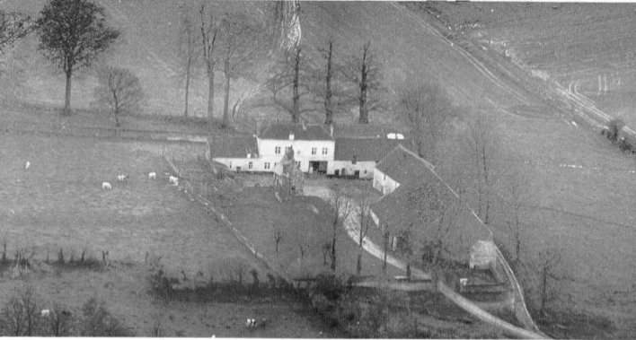
16. Hougoumont. The ruins of the chapel are in the courtyard; the south garden wall centre left.
